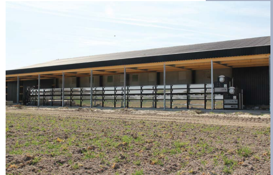
Manure drying with ventilation air from the poultry house
